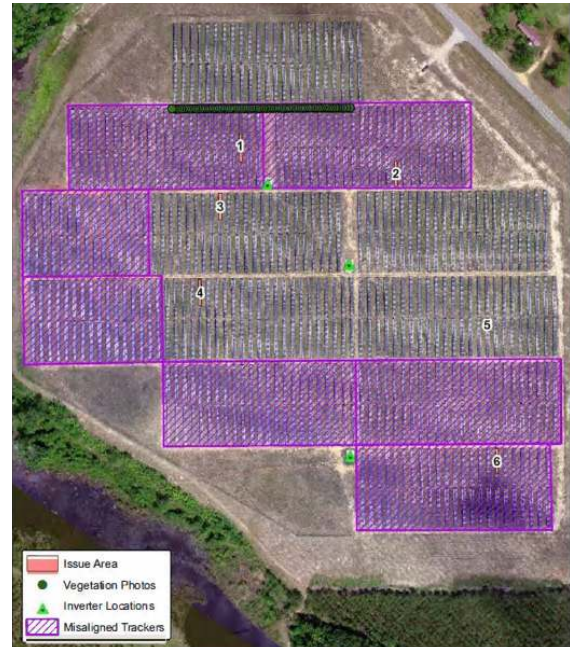
Fig. 3.1 Inspection Overview. Visual orthomosaic displaying key site features and issues identified. This image was created via georeferenced imagery collected by drone flyover and later stitched together into a single site overview.
