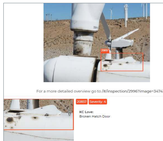
Figure 4.3 Sample wind inspection report results.
