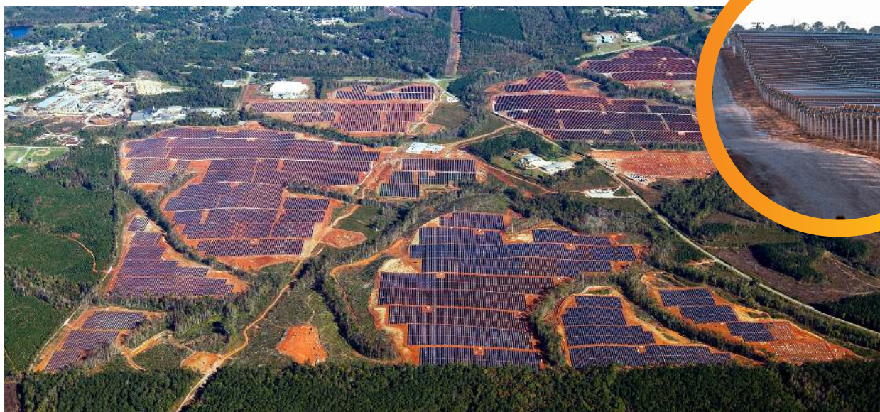
Actual site with integrated TrueCapture. Location: Lafayette, Alabama.
